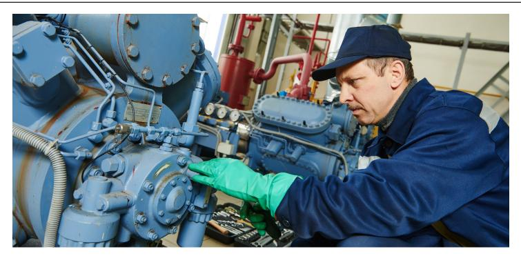
In studies it has been identified that excess oil in refrigerant will cause a significant degradation in performance. Chiller manufacturers recommend levels no higher than 0.5%. However, it is not uncommon for excess oil to build up at levels ranging from 3%–9%.
